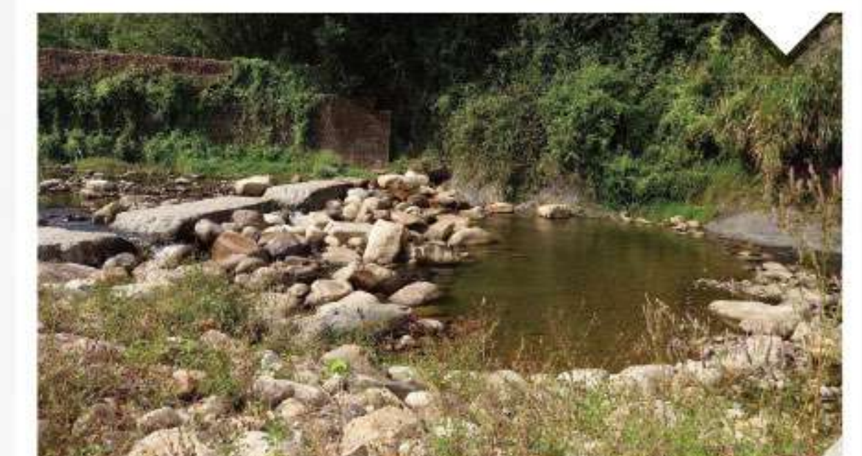
Reconstructed weir, now friendly to aquatic organisms, and bottom left, rocky plant covered bank that was previously a concrete wall four meters high.
