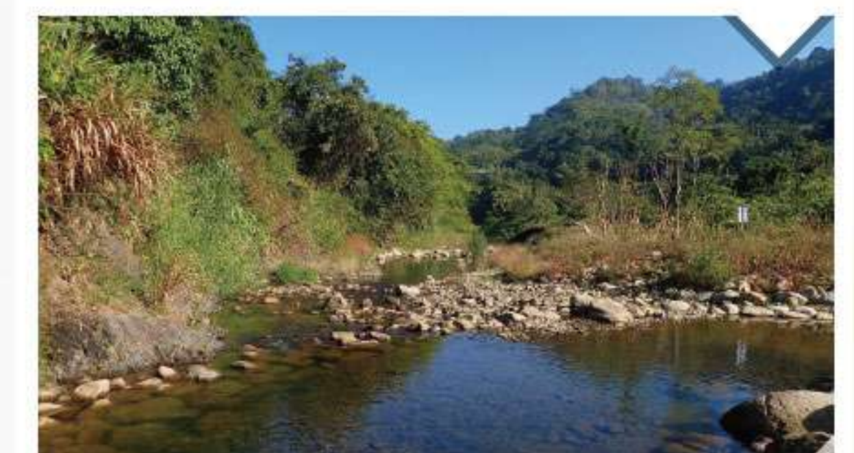
The recreated natural stream structure with pools, riffles and sloping vegetated banks.
