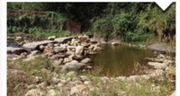
Reconstructed weir, now friendly to aquatic organisms, and bottom left, rocky plant covered bank that was previously a concrete wall four meters high.
