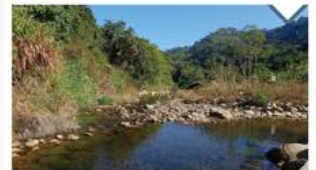
The recreated natural stream structure with pools, riffles and sloping vegetated banks.
