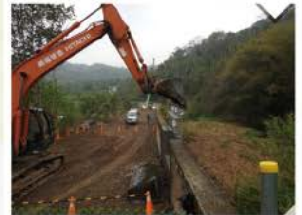
The wall starts coming down, March 2023.
